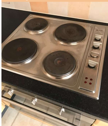
Rust signs on hob
